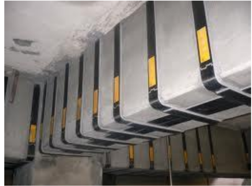
Strengthening of Shear
