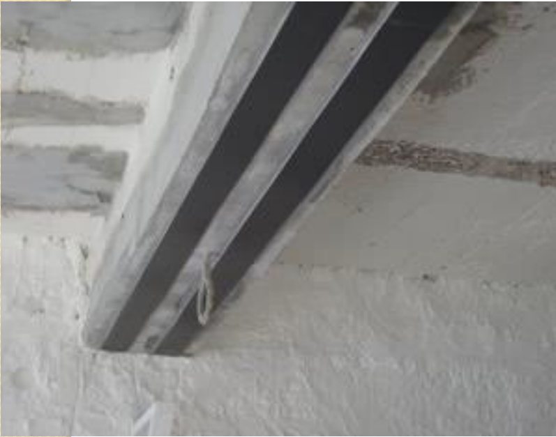
Strengthening of Flexure
