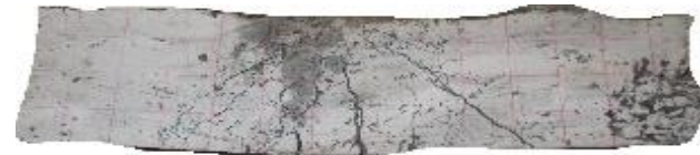
b) T=300^{\circ}\text{C} (flexural failure)
