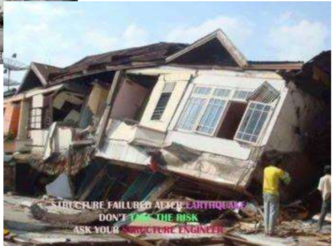
COLLAPSE DUE TO SOFT-STOREY E
