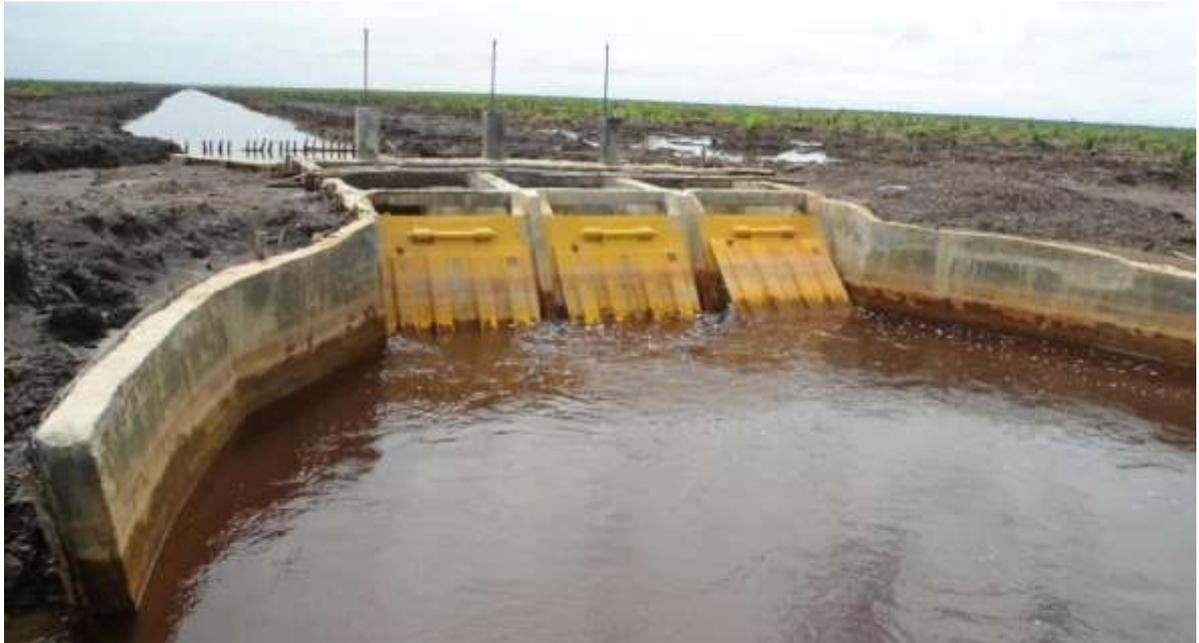
Gambar 2.7. Pintu Air Tipe Flap (Sumber : Anonim, 2013)
