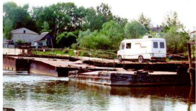
Figure1. Pontoon foundation with bridge decks
