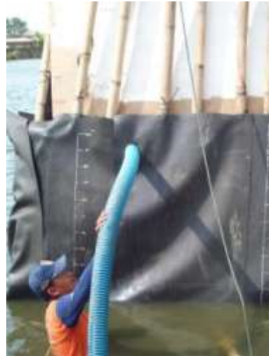
Figure 6. The sinking process of pontoon [10]
