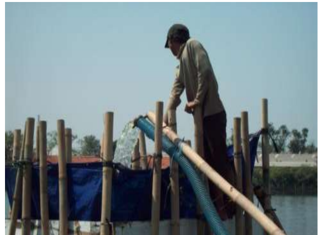
Figure 8. The Loading process of pontoon[10]
