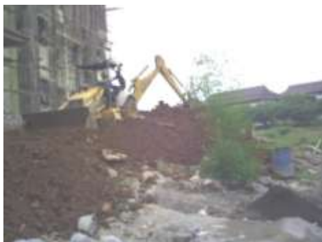
Figure 3 Landfill construction after the start of building construction
