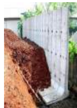
c) Retaining wall
